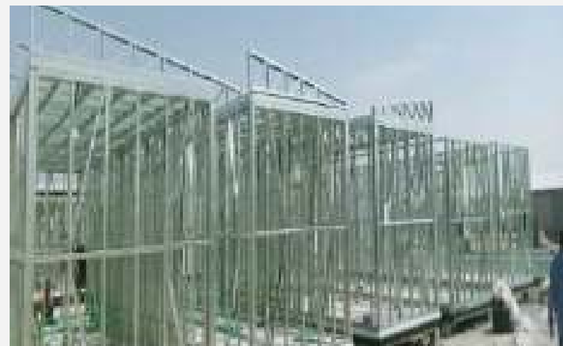
04 Pre-assembly at Shop
